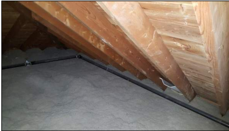
Photograph 2: Attic insulation and insulation baffles (West Wing)
