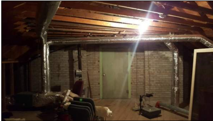
Photograph 3: Attic separation wall (East Wing)
