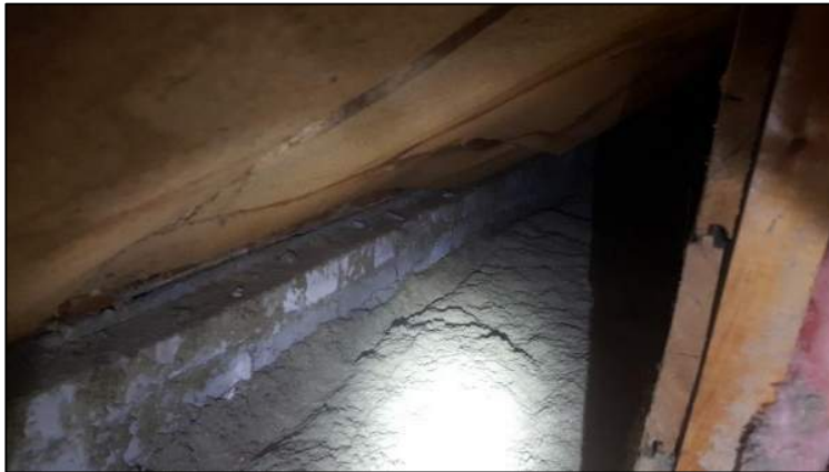
Photograph 8: Roof space in front of dormer
