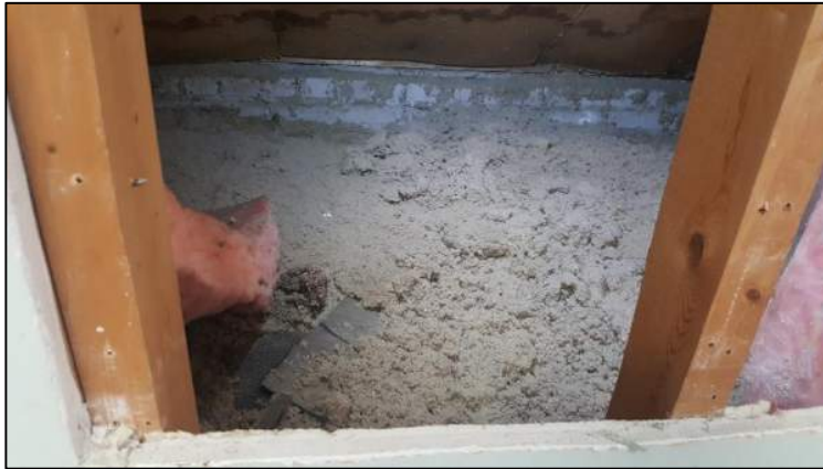
Photograph 7: Roof space between dormers
