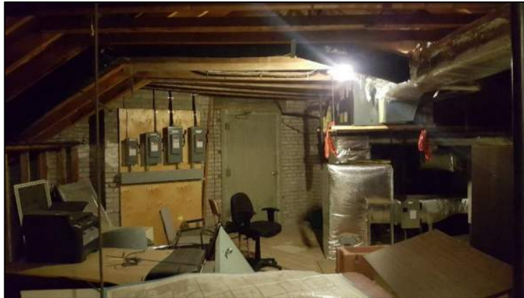
Photograph 1: Attic separation wall (West Wing)
