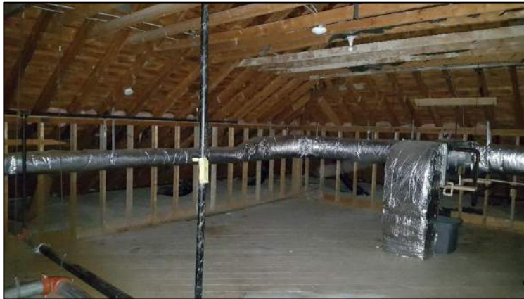
Photograph 4: Attic framing and perimeter insulation
