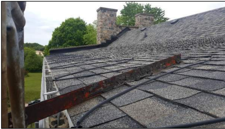
Photograph 5: Low slope roof
