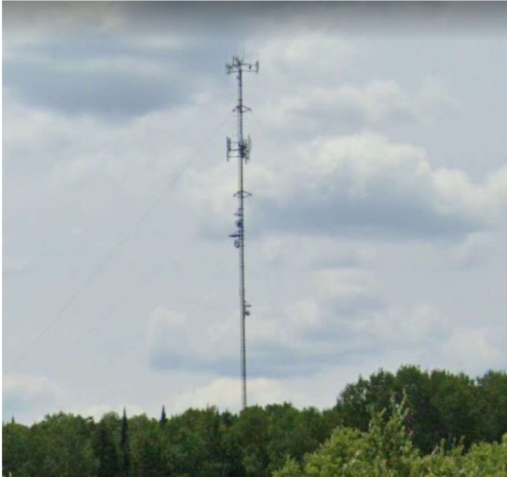
Figure 3: Google Street View image of the tower located within the subject land. The image was taken from Highway 520, looking east
